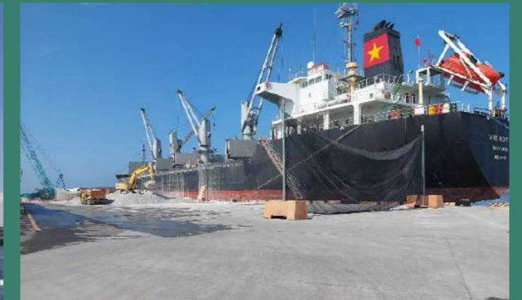
Dust Control Nets Installed for Loading and Unloading Operations
