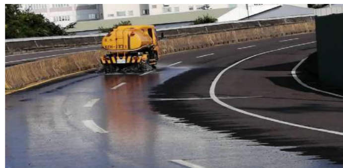
Using Reclaimed Water for Road Cleaning to Prevent Dust Emission
