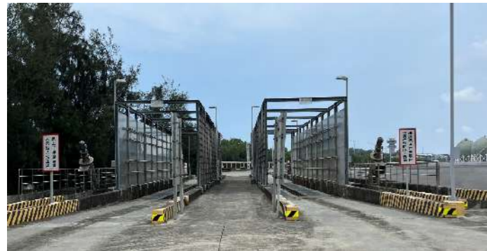
Car wash tank
