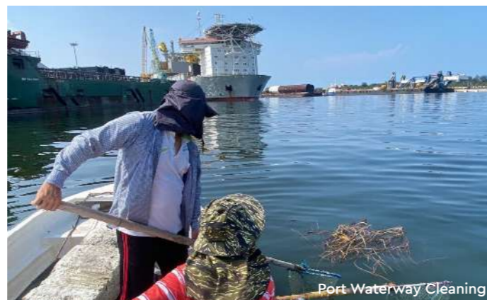
Port Waterway Cleaning
