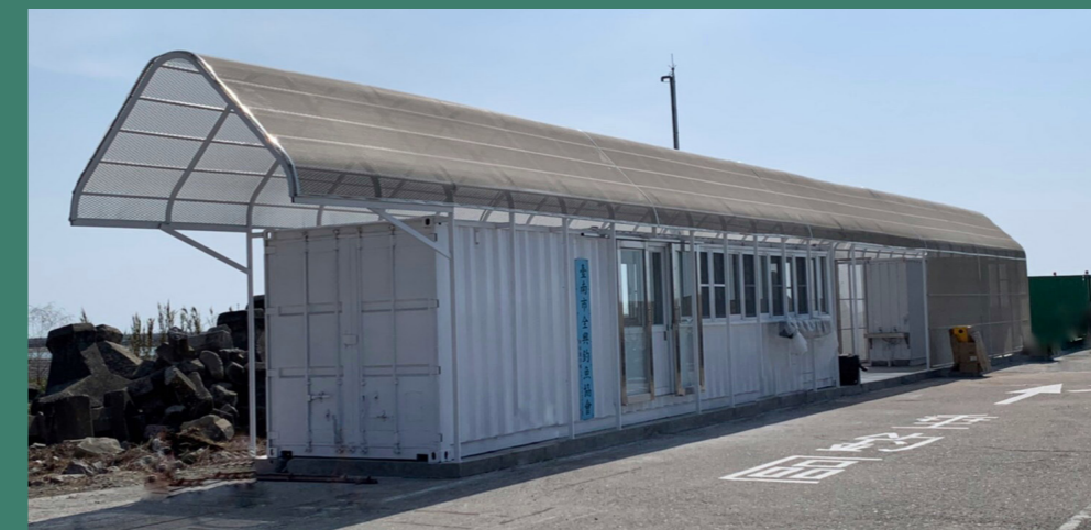
North Breakwater Fishing Area Management Station and Toilets
