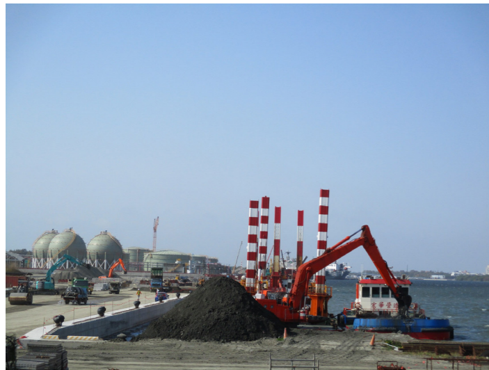
Dredging at Dock 17, 18
