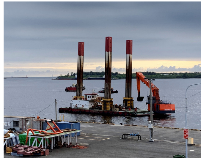
Port area dredging
