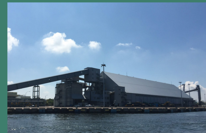
Automatic coal unloader and enclosed coal warehouse
