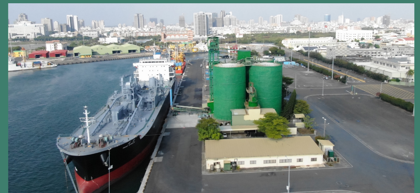
Pipeline transportation and enclosed warehouse are used for cement loading and unloading to reduce dust.
