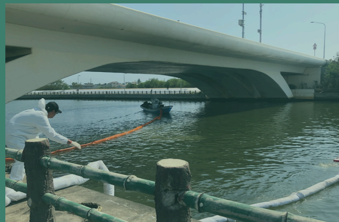
Laying oil-absorbing cotton and oil-retaining rope
