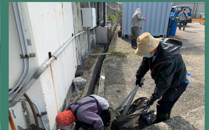
Cleaning and mantainese work for port
