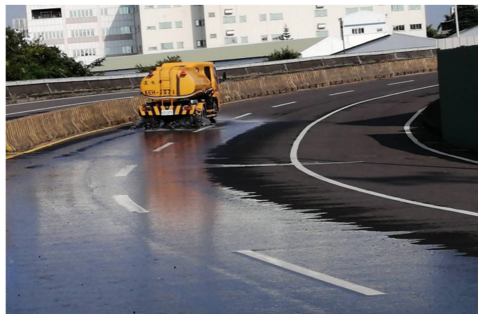
Road cleaning to avoid dust
