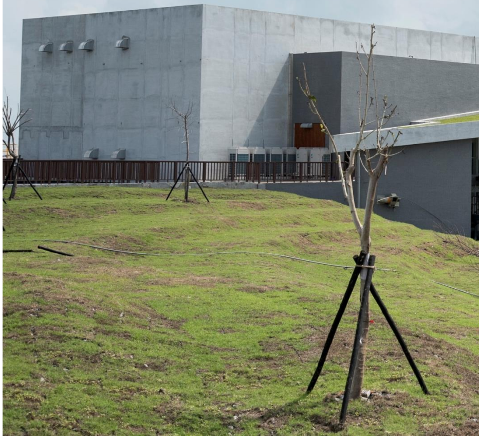
Wastewater Treatment Facilities
